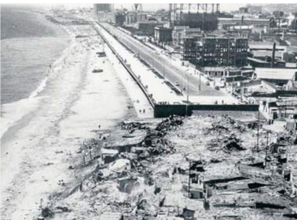
HOSPITAL DEL MAR
